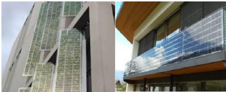
Figure 8: BIPV systems on external integrated devices [20]
