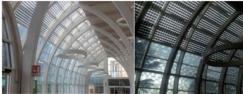
Figure 9: PV glass tower of the Meier Hospital [21]
