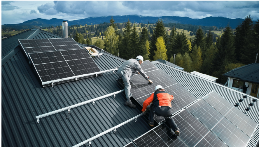
Figure 2: Example of Work Activities During Photovoltaic System Installation
