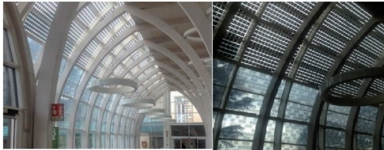
Figure 9: PV glass tower of the Meier Hospital [21]
